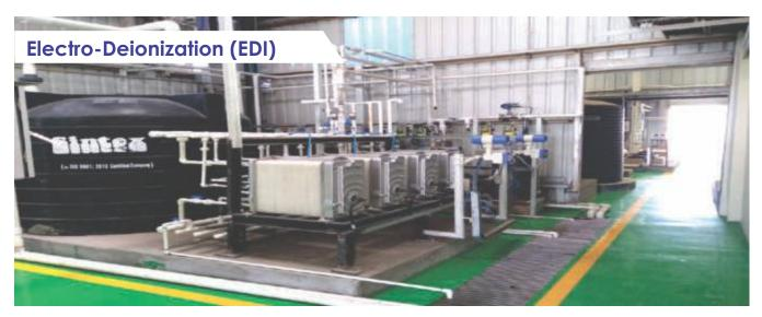
Electrodialysis is a process in which electrically charged membranes are used to separate ions from aqueous solutions under the driving force of an electrical potential difference. Because of the arrangement of ion-selective membranes, the migrating ions become concentrated in each alternate cell in the stack.
