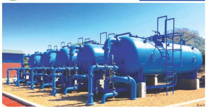
We offer series of filters like Vertical & Horizontal Pressure Sand Filter, Activate Carbon Filter, Dual Media Filter, Iron Removal Filter in different sizes at a low cost, reliable and efficient way to filter impure water. It consists of different grades of sand, Activated Carbon, Anthracite, MnO2 as per application. This plant Removal of suspended solids and turbidity, color and free chlorine in less quantity
