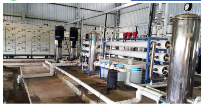
Reverse Osmosis system are designed and manufactured to remove total dissolve solids (TDS) from raw water. We are using advance membrane technology in our RO's to allow water to pass through a semipermeable membrane.
